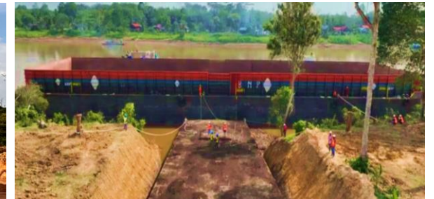
Physical test of jetty for manual loading
