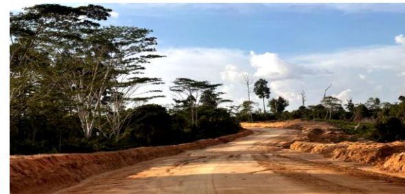
Portion of completed hauling road
