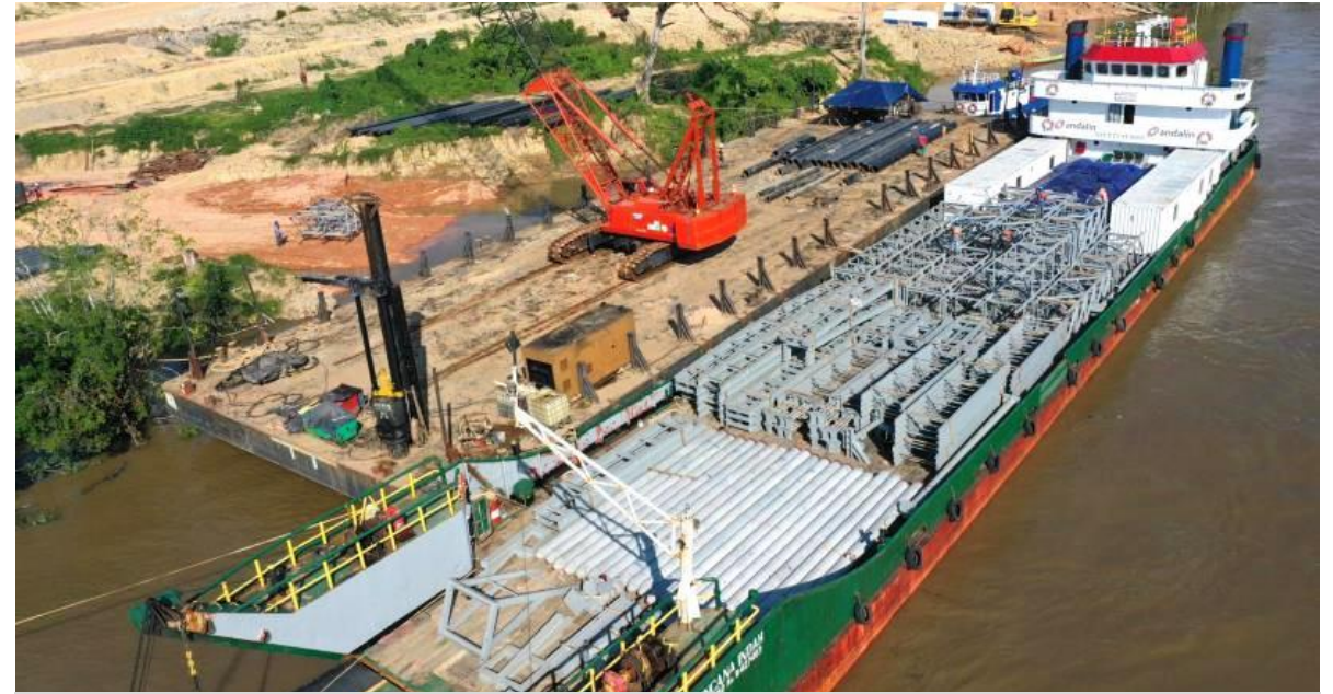
Material delivery for conveyor construction
